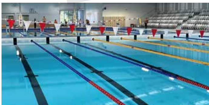
50m Pool with Moveable Bulkhead
